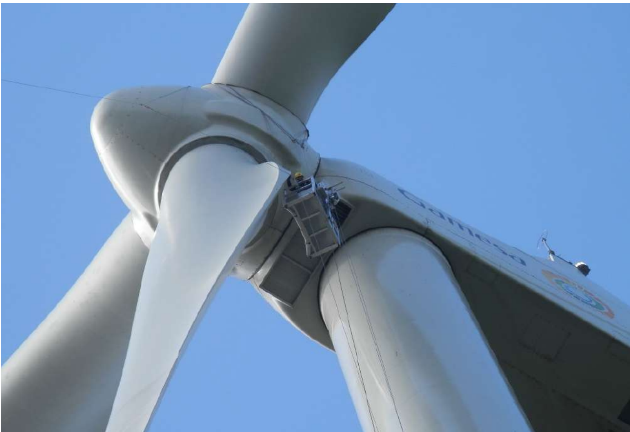
GAMESA G10X, blade maintenance (output edge access)
