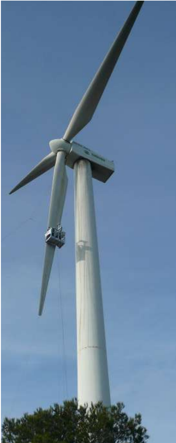
GAMESA G4X y G5X, blade maintenance (fiber)
