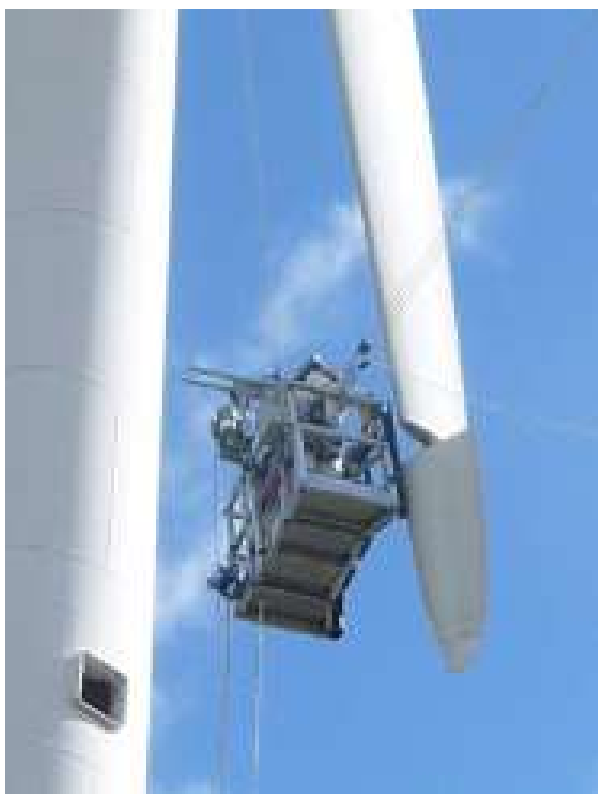
MADE, blade maintenance (end)
