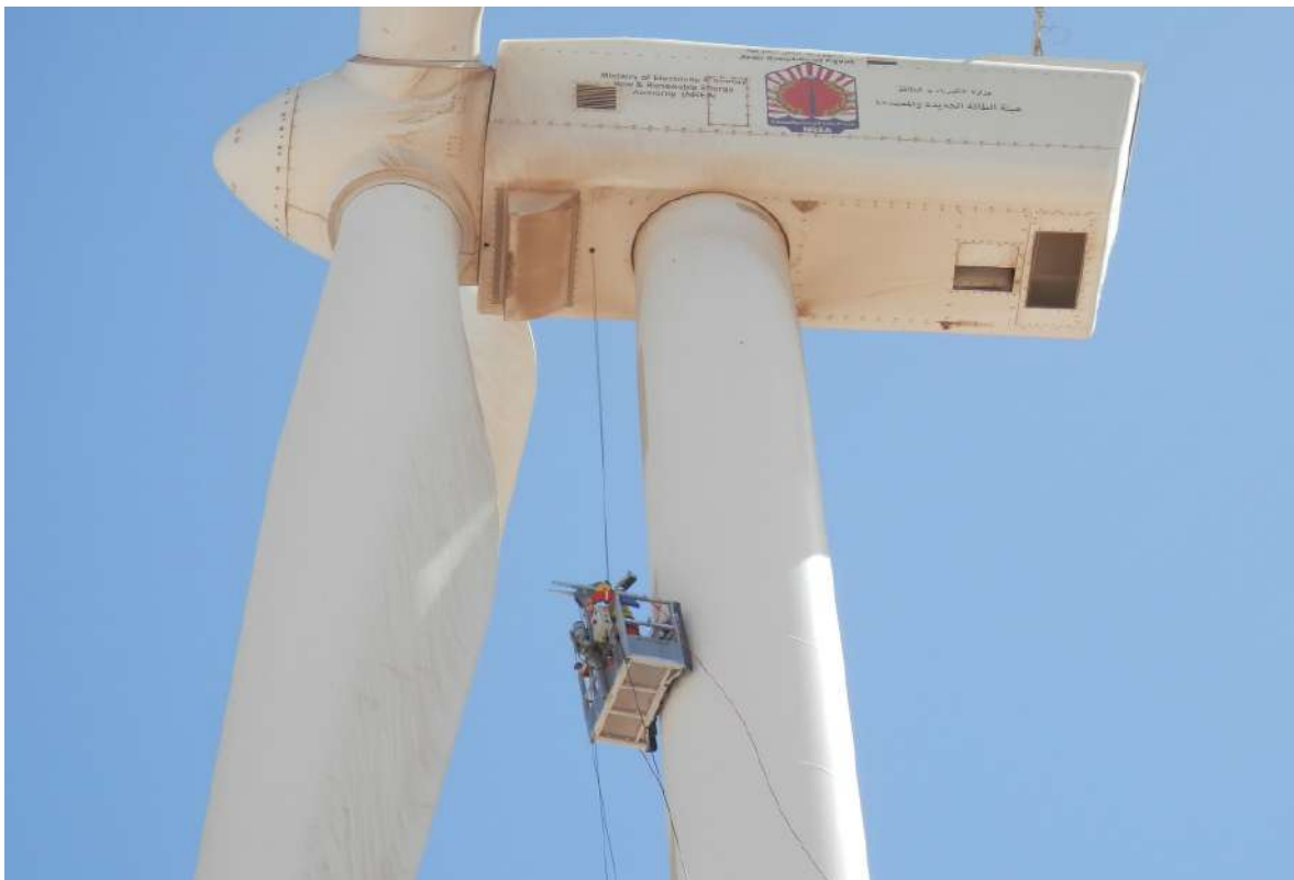
GAMESA G8X, tower maintenance (cleaning)
