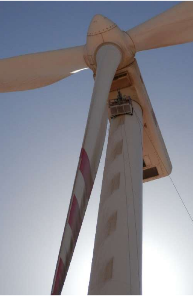
GAMESA G8X, tower maintenance (cleaning)
