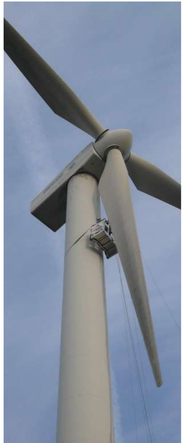
GAMESA G4X y G5X, tower maintenance (cleaning)
