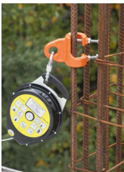
Real-life applications of the temporary anchor point for PAT 187 formwork bars.
