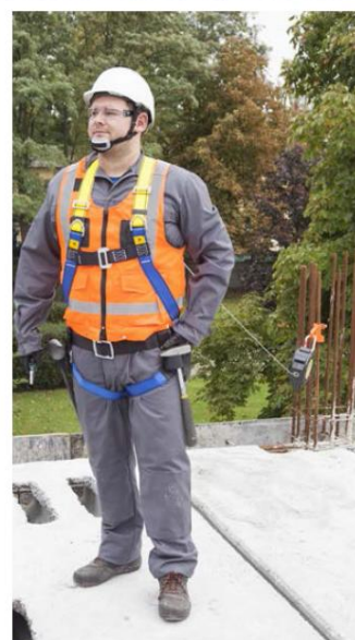
Real-life applications of the temporary anchor point for PAT 187 formwork bars.
